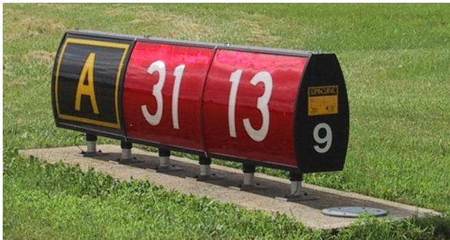
Fig. 9 Runway Holding Position Sign
