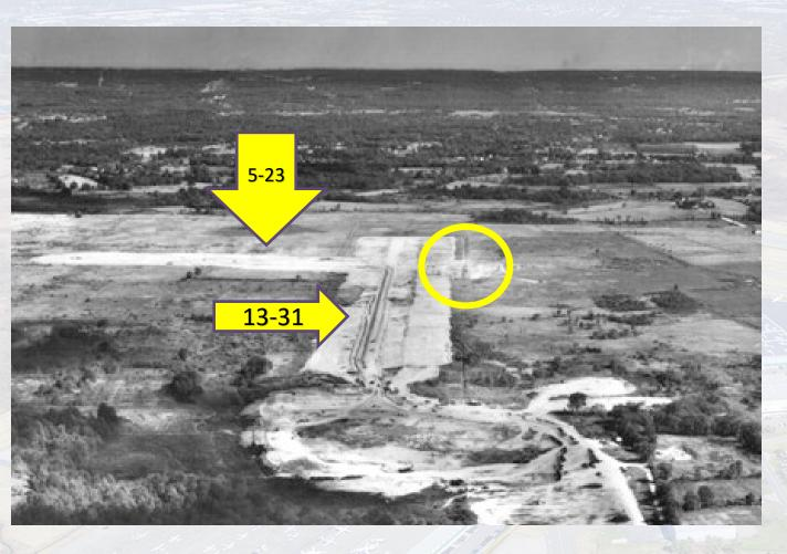
As part of the original development of Morristown Airport, a 36-inch drainage pipe was installed in order to allow water flow underneath Runway 5-23.
