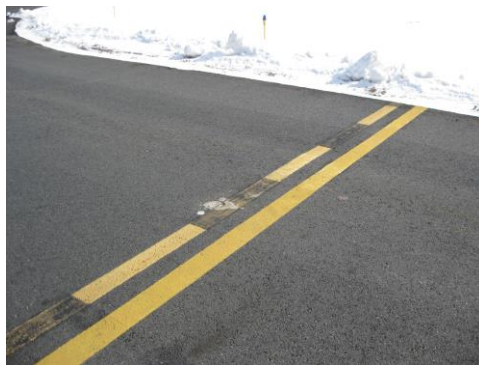
Fig. 6 Non-Movement Area Boundary Marking
